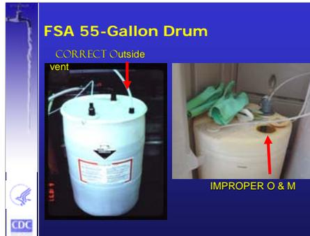
A common delivery mode for FSA is a 55-gallon drum. These have been used as day tanks in some cases but normally should not be used in such a fashion. A properly sized tank made for that purpose should be used instead. This polyethylene tank shows that a tank can be easily vented with a flexible hose. The second photograph demonstrates corrosion in the vicinity of an incorrectly vented tank.
