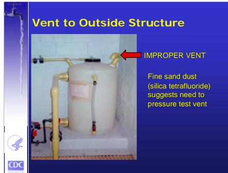
This tank is not correctly vented to the outside. Ensure that the tank is sealed and vented to the outside and that it does not release within the building. This installation will experience corrosion problems within the building.
